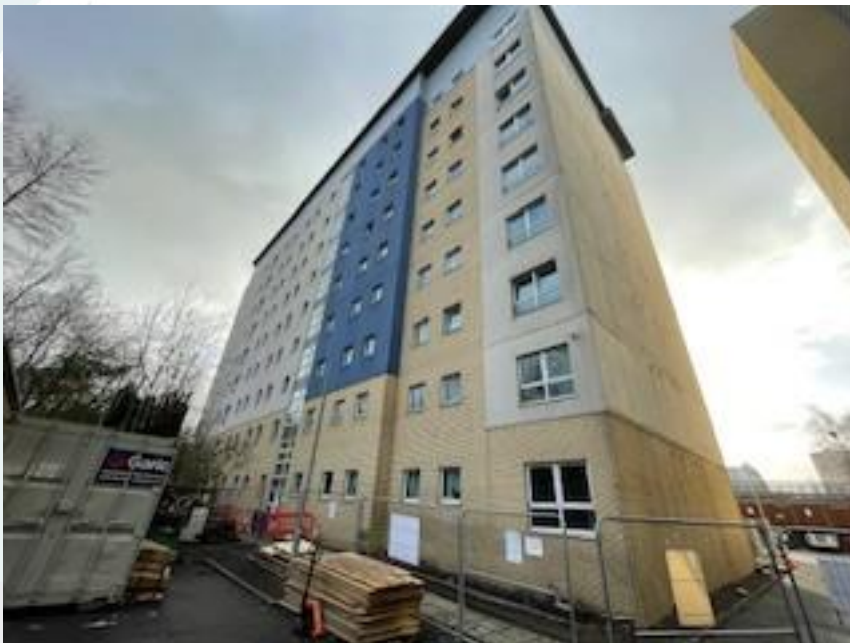
Phase 4 scaffolding will commence
